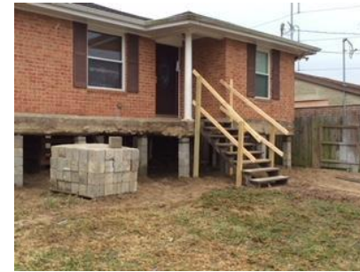
Figure 7. Temporary Cribbing
